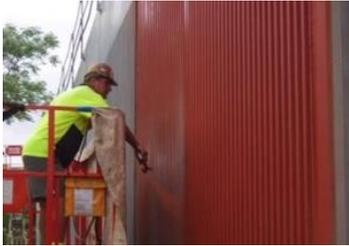
Inorganic silicate concrete coating specifically formulated to form an extremely strong permanent chemical bond with concrete substrates. COATING version designed to be thicker with better hiding for use as a top coat. Application is similar to conventional coatings but ingredients in **COATING CoSi** are designed to react with lime in concrete to form an extremely strong bond resulting in a superior, very durable, extremely tough, permanent protective coating.
